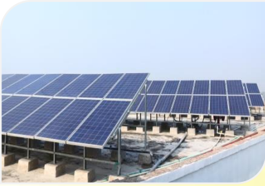
1. Solar generation Installation of Solar panels
